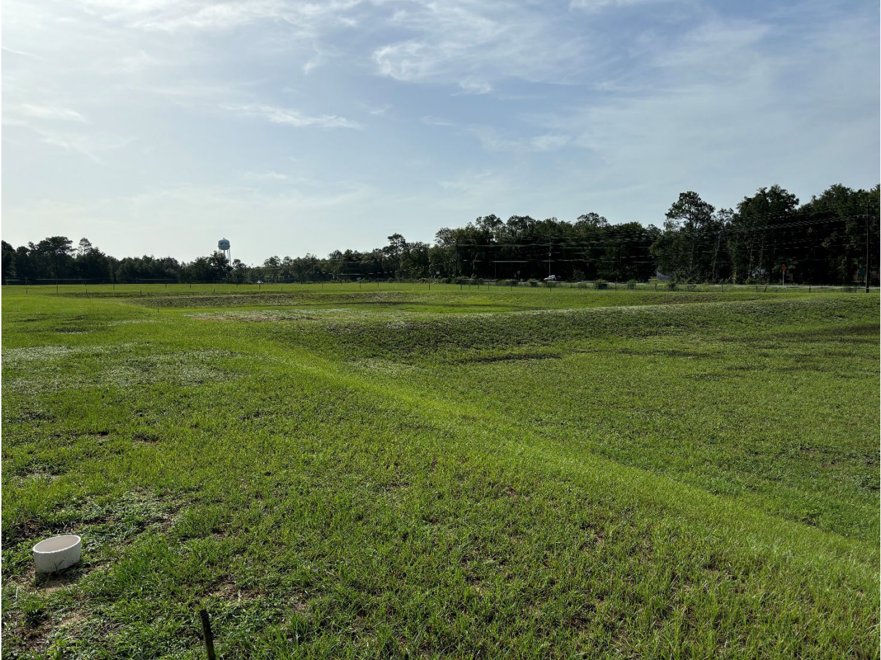
Figure 3.7 - Infiltration Basins at the Existing WWTF in Bronson
