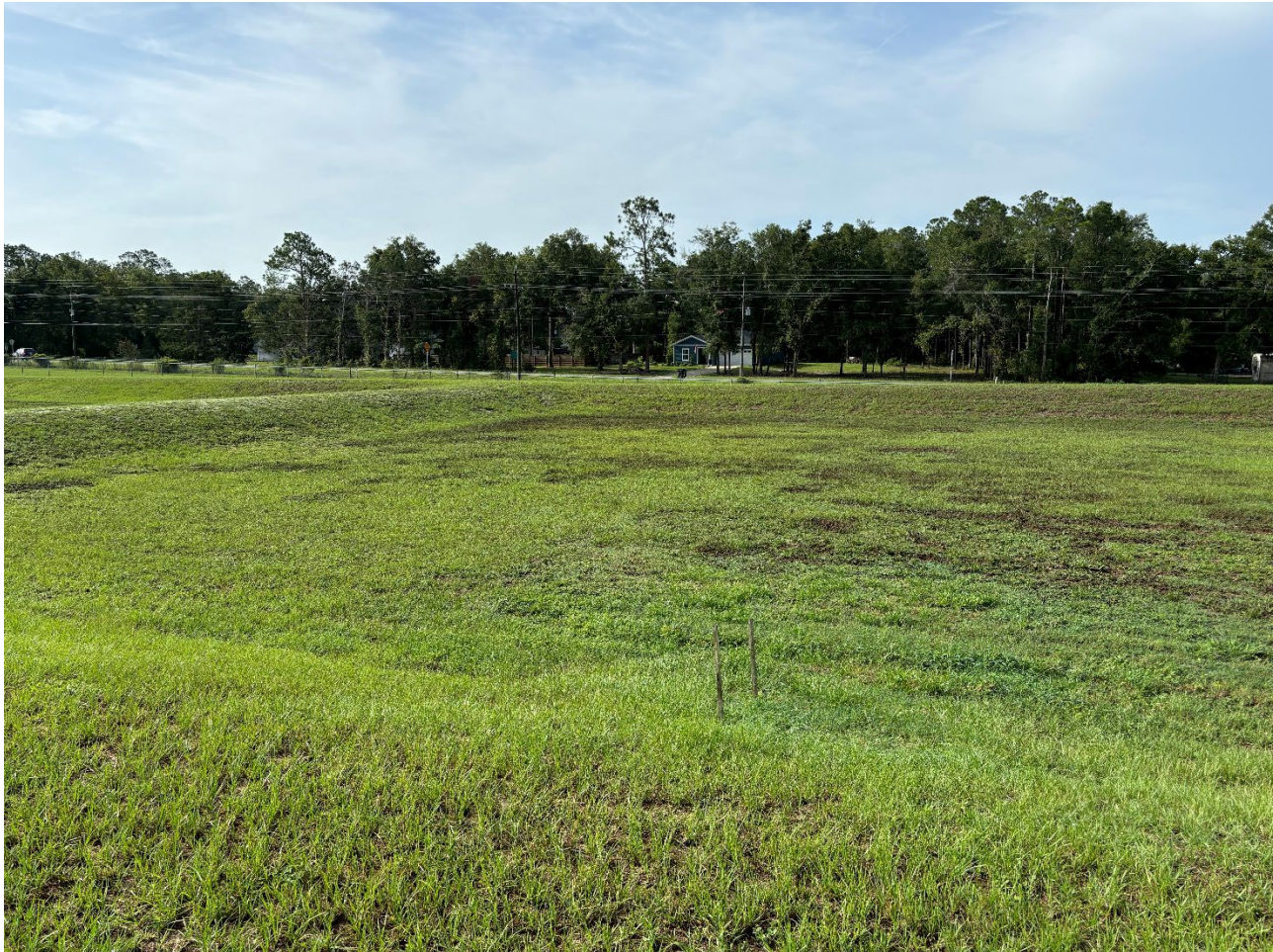
Figure 3.8 - Infiltration Basins at the existing WWTF in Bronson
