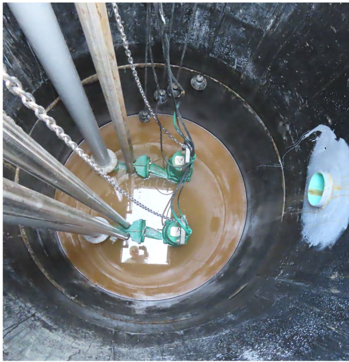
Pump Station-Wet Well
