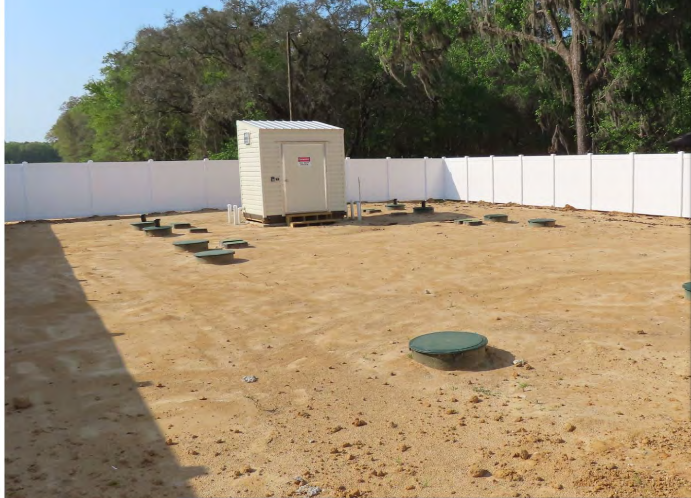
DWTU tanks installed w/ controls building and fencing
